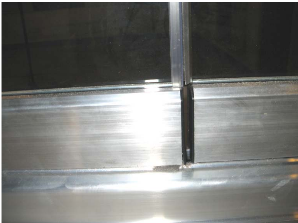
Fig. 4: View Receiving Room, Measurement 2, Detail
